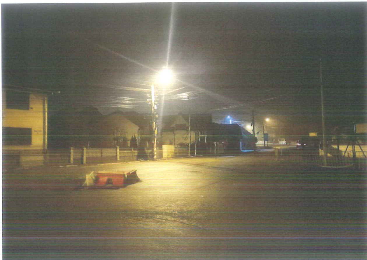
Laminoristilor-lampi defecte, stilp fara lampa iluminat neuniform
