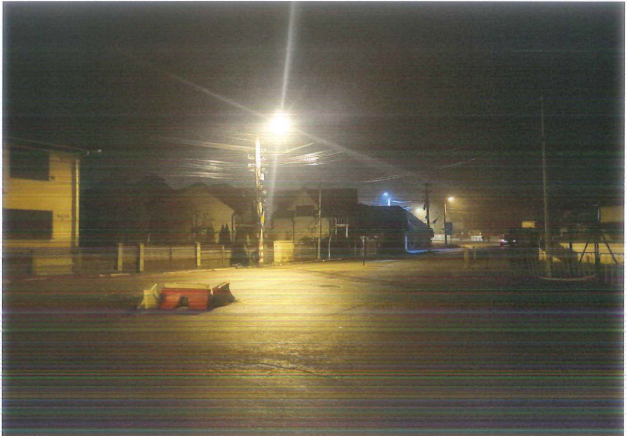
Laminoristilor-lampi defecte, stilp fara lampa iluminat neuniform
